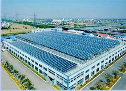
Figure 8: Installation of 7 460 m 2 of ETC in a printing and dyeing plant in China
