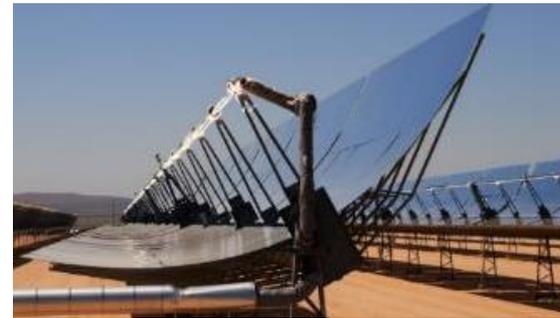
Parabolic Trough Collector - PTC
