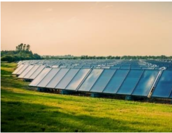
Flat Plate Collector - FPC
